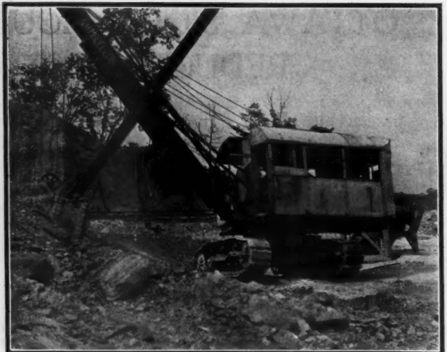
Shovel Stripping Overburden
